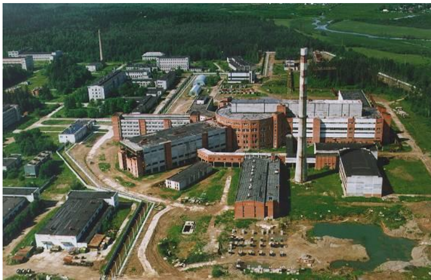
FIG. 1. The general view of the PIK reactor site.
